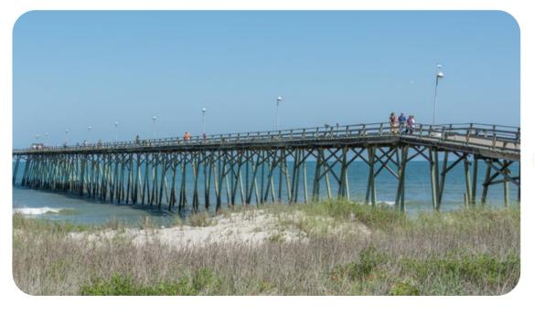
Bertha caused so much damage the pier had to be reconstructed, the new owner returning to the original design including an impressive 26-feet elevation. The added height seems to have helped in later storms with little damage since.
